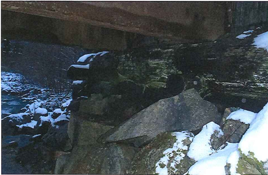
CK2087 Right Abutment
